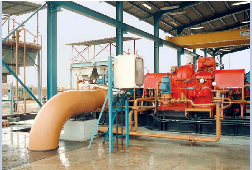
Variable-speed turbo coupling type SVL in a pipeline pump drive.
